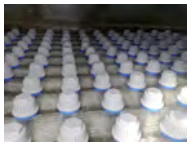
Nozzles plate according DIN 19643/ÖNORM 6216
