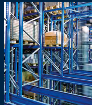
Fully automatic high rack systems for quick delivery
